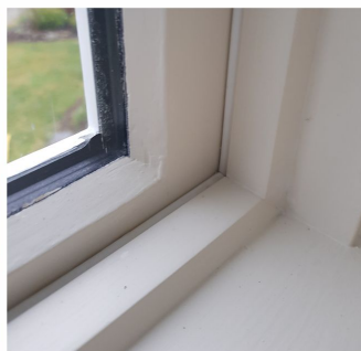
Paint Finish Air Seals
