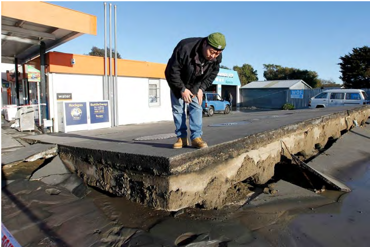
Figure 6 Fuel tanks have buoyed up through the ground surface as a result of liquefaction of the enclosing sediment, .Christchurch area, February 2011. Photo: R.D. Beetham, GNS Science.
